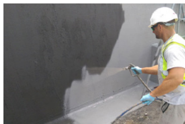
APPLICATION OF ACRYLIC & CEMENTITIOUS WATERPROOFING PRODUCTS
