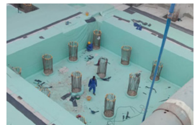
PILE HEAD TREATMENT (FOR PVC)
