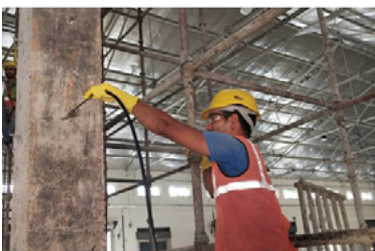
REPAIRING WORK, INJECTION WORK
