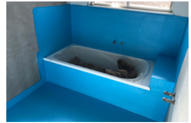
WET AREA WATERPROOFING WITH THE CEMENTITIOUS, RUBBERIZED, POLYURETHANE.
