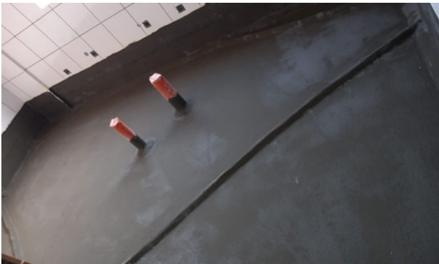
RUBBERIZED BITUMEN COATING
