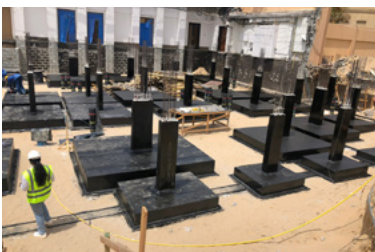
SUBSTRUCTURE WATERPROOFING (APPLICATION OF TROCH APPLIED, COLD APPLIED & SELF-ADHESIVE MEMBRANE)
